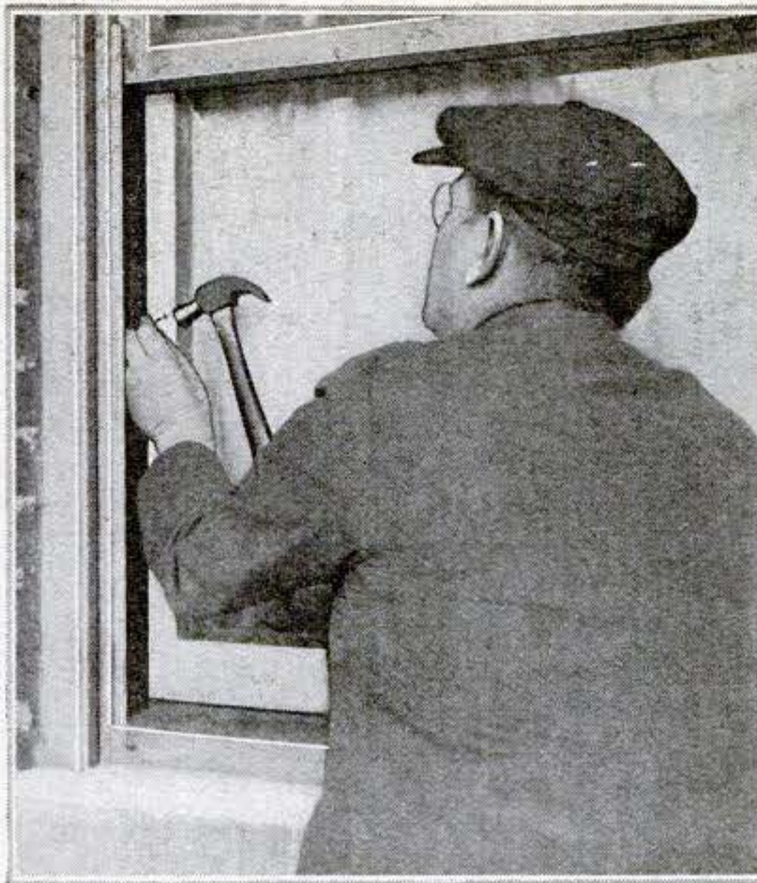
Examine the nails around your window-casing: if any have become loose, you will save coal by tightening them
