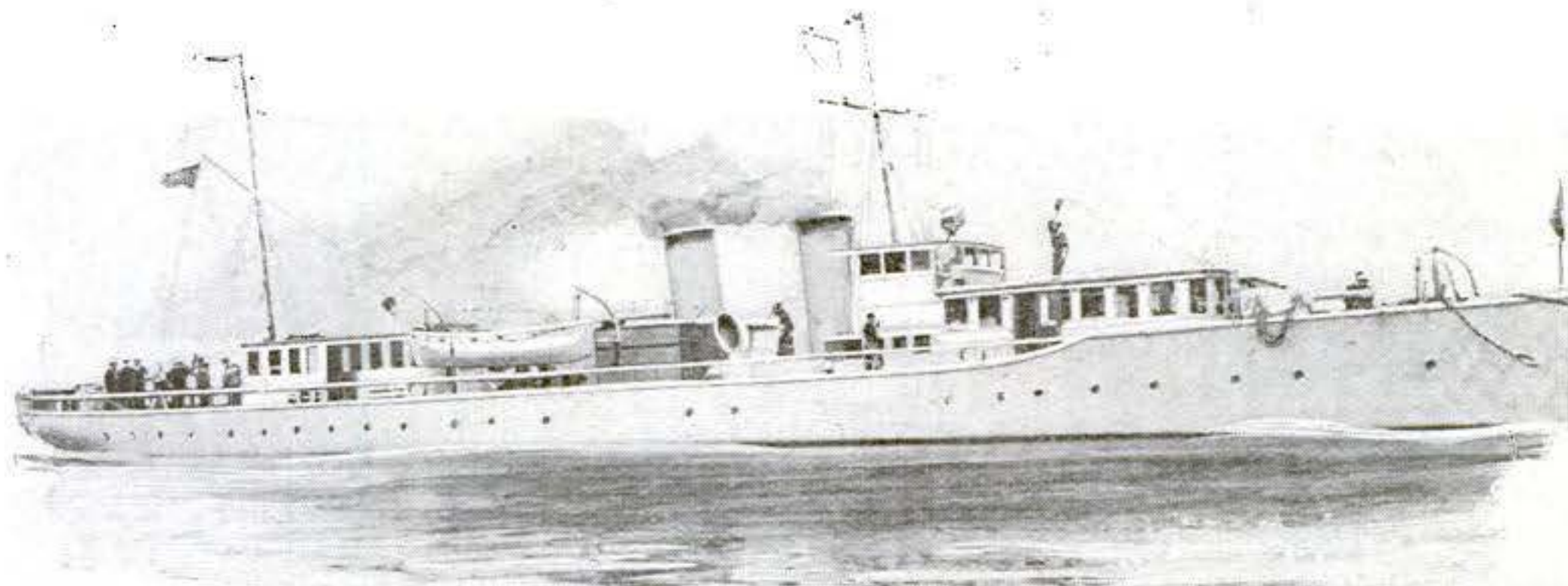
The U. S. S. Gem, which has been used to test different types of fuel; she has made many successful trips operating on pulverized coal
