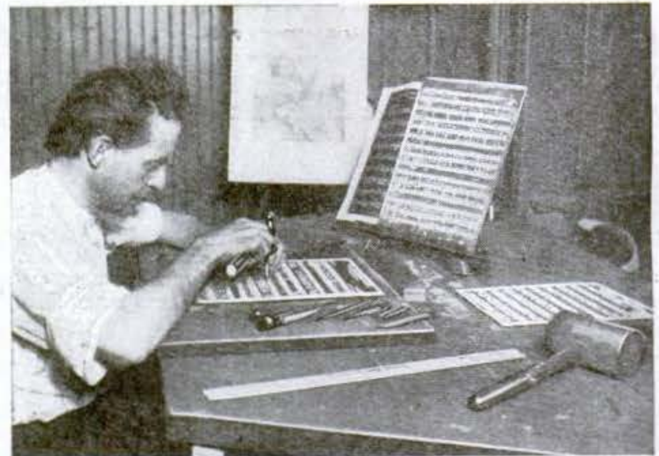
The notes are very hard to etch; so, after the acid bath, they are hammered in by an expert
