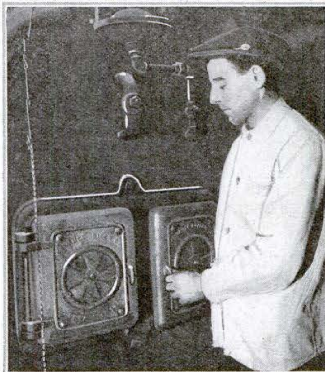
If the air enters from below, in burning soft coal, the oxygen is burned out; the remedy is to let in air from above
