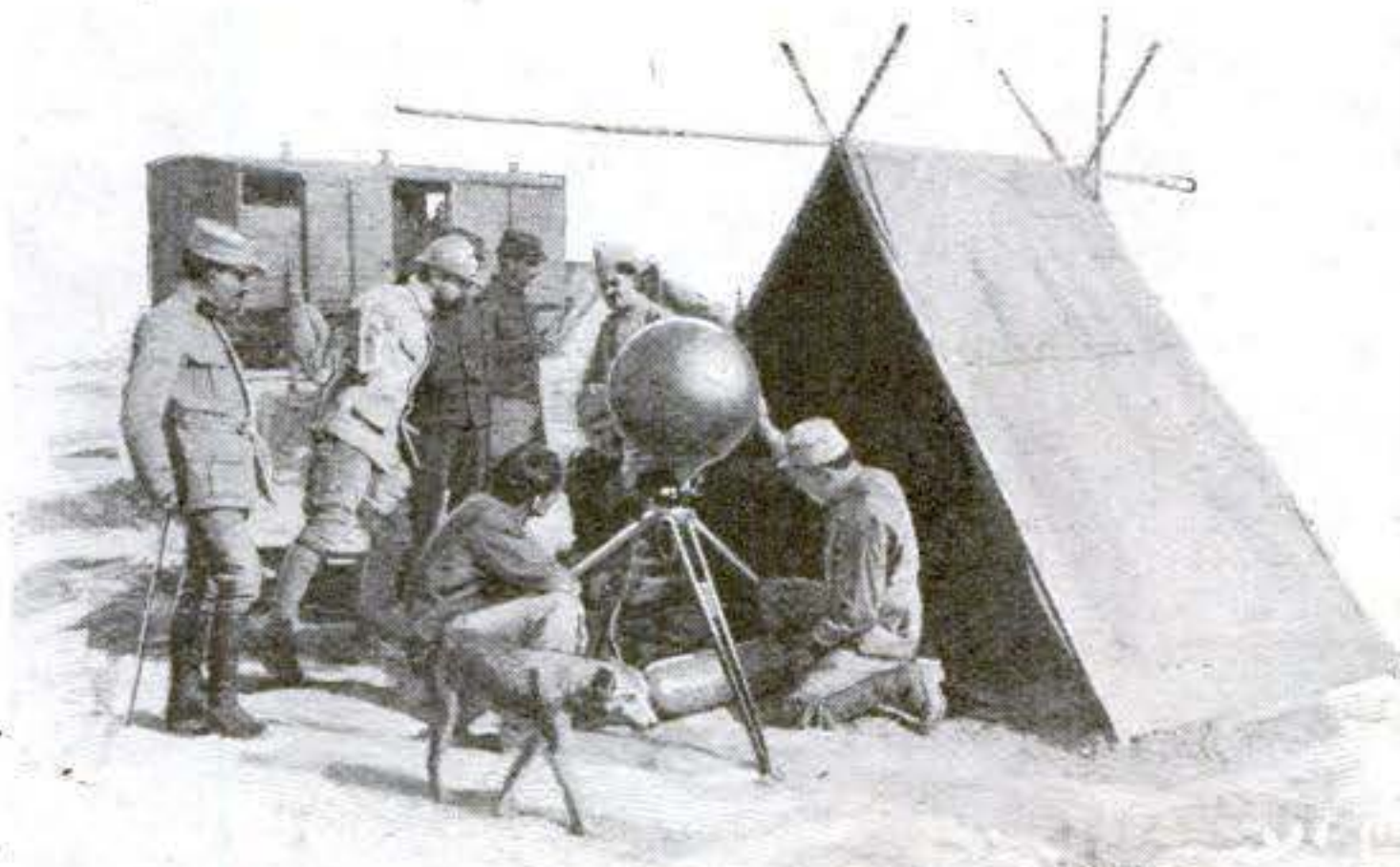
When the balloon ascends, its course is watched to learn the wind's velocity and direction
