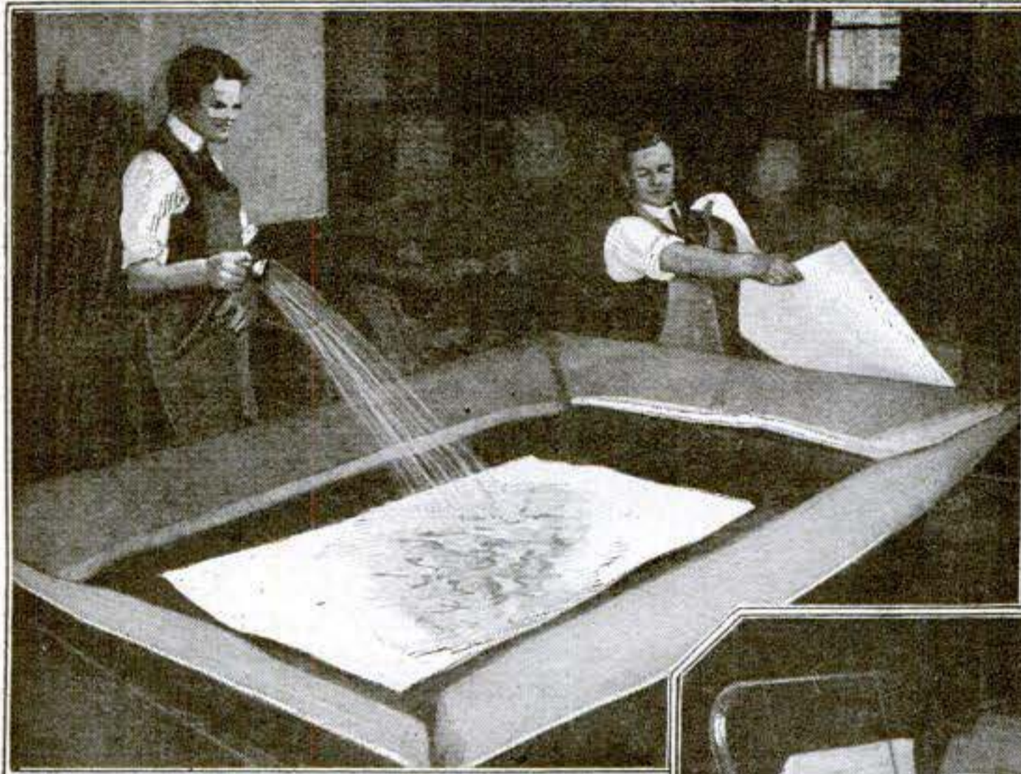
Before the sheets of manila paper are run through the press to be embossed they are sprayed with water. Because of the great strain it must bear, only paper of a very tough quality can be used
